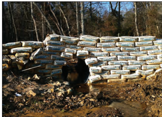
Figure 8.22. Sacks of concrete used to stabilize fill.
