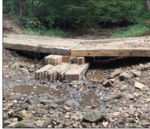
Figure 8.3. Crane mats installed over an ephemeral channel on a haul road.
