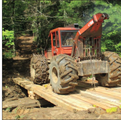
Figure 8.4. Crane mats used for skidding across a perennial stream. Note intermediate span support.
