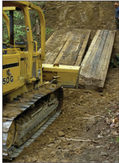
Figure 8.1. Three panel wooden skidder bridge installation.
