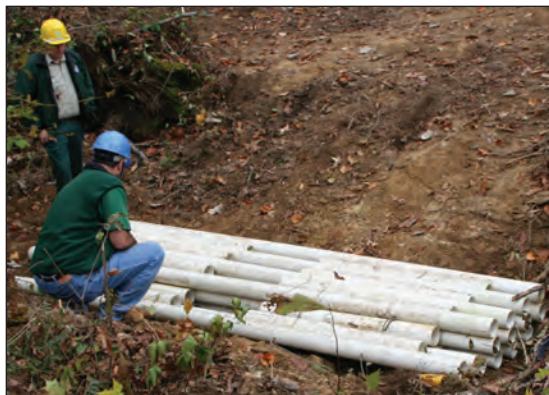
Figure 8.8. PVC pipe bundle installed in ephemeral channel, folded over itself to ensure channel bed is covered and top pipe layer is flat across the top.
