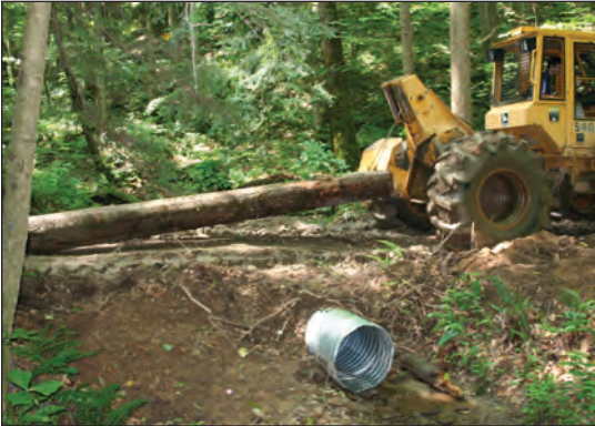
Figure 8.12. Culverts are one of the most common crossings used for skidding and hauling.
