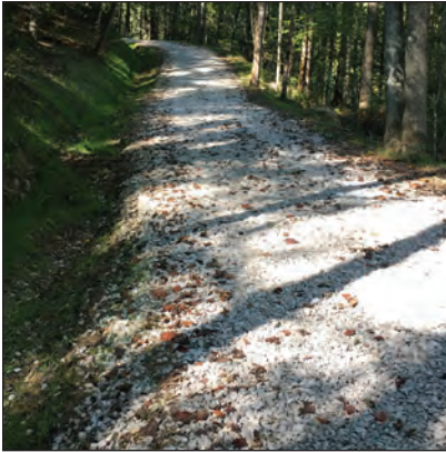
Figure 9.8. A well-constructed haul road, with gravel in-sloped surface and seeded ditch.
