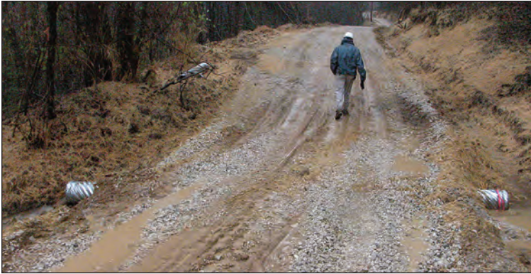
Figure 9.12. Corrugated steel culvert used to cross drain the ditch on an in-sloped haul road.
