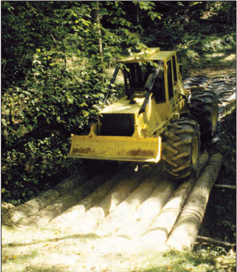
Figure 8.5. Log bridge developed using recommended lashing design.
