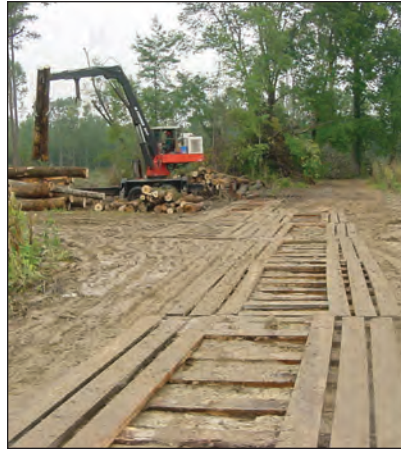
Figure 9.16. Wooden mats, made specifically for logging or for use in construction can be effectively used for haul road protection.
