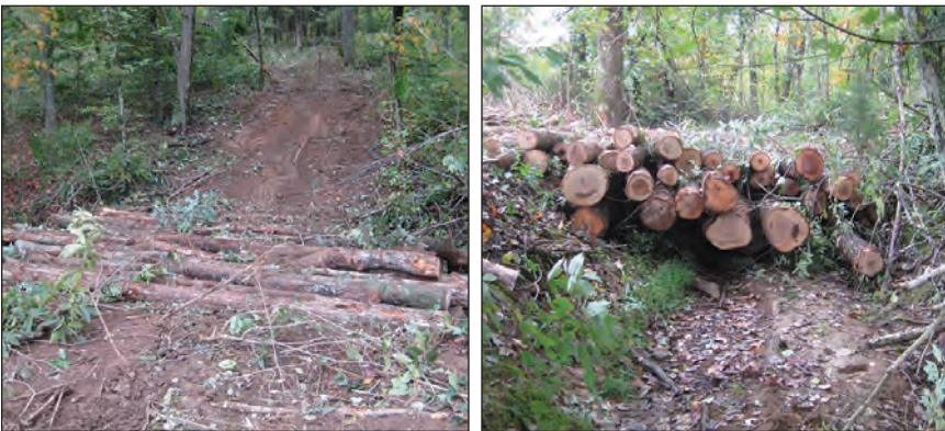
Figure 8.17. Pole crossing used for skidding across an ephemeral channel during the dry season.
